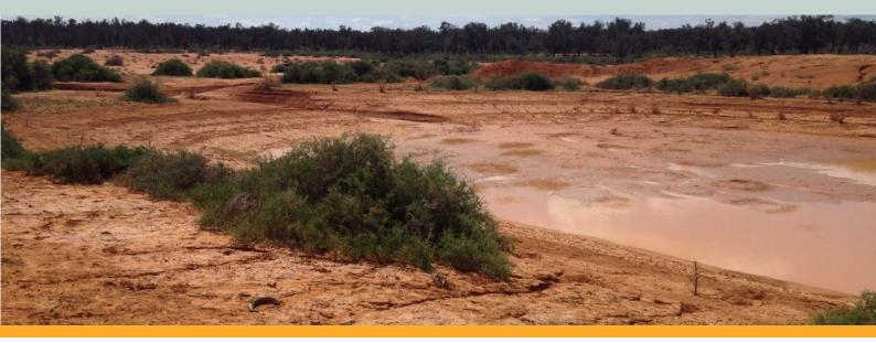
Figure 4: Water entering the silt trap and settling before it is pumped to the Superdam.
