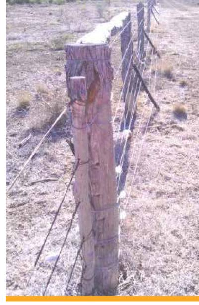
Figure 2: The electrified boundary fence with 3-wire off-sets, positioned 45 degrees to the fence to reduce invasion of wild dogs.
