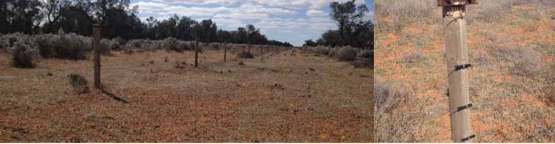
Figure 2: Second-hand vineyard posts used as fence posts.
