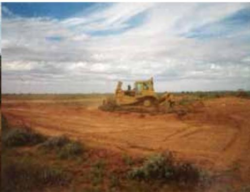
**This is the same area once the machinery were engaged at the 'Drug Creek Site'. The gully system was flattened to produce a good platform for the bank to be built.**
