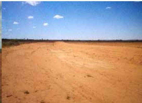
**The first of five banks was built on the site. The first bank needed to be 'chunky' to take the first hit of storm flows of water. The other banks were smaller, and also cheaper to develop. Images taken in 2011.**
